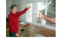
9. Place the wet adhesive side of the film onto the glass.
