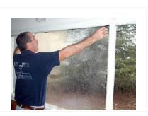
3. Cut the film to the size of the window, leaving ¾" (2 cm) overlapping edges all around. Alternatively, measure the window and pre-cut film out of the box or on a Film Handler.
