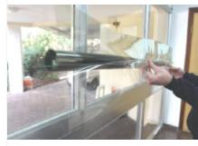
2. Spray both sides of the exposed 6 inches with the wetting solution.
