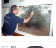
14. Wet the film surface again, and pressing hard with the squeegee, wipe out from the center until all the air bubbles and remaining water have been removed from the edges.
